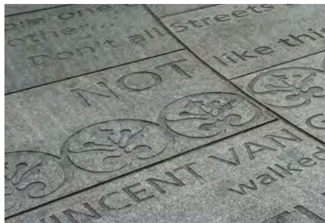
Utilizing permanent infrastructure for path infrastructure
