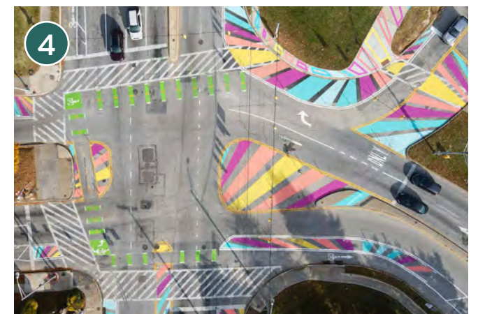
Intersection improvements near Lake Montebello
